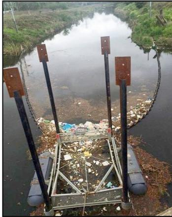
▲ Weighing in at 1.5 tonnes, installation of Mobile's 30' x 13' litter trap at the mouth of Eslava Creek has commenced. Paddles direct surface litter into two wire mesh basket traps that require vigilant emptying. Its \$660,000 ticket price is worth it to city officials. "It's not the answer but part of it," said one.
