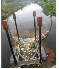
Weighing in at 1.5 tonnes, installation of Mobile's 30' x 13' litter trap at the mouth of Eslava Creek has commenced. Paddles direct surface litter into two wire mesh basket traps that require vigilant emptying. Its \$660,000 ticket price is worth it to city officials. "It's not the answer but part of it," said one.
